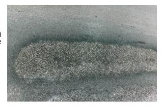
8. The cut of the road damage repaired with the technology of Blow Patching
